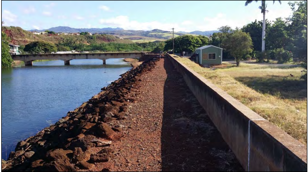
Figure 52. SIHP # -2283, floodwall, view to north
