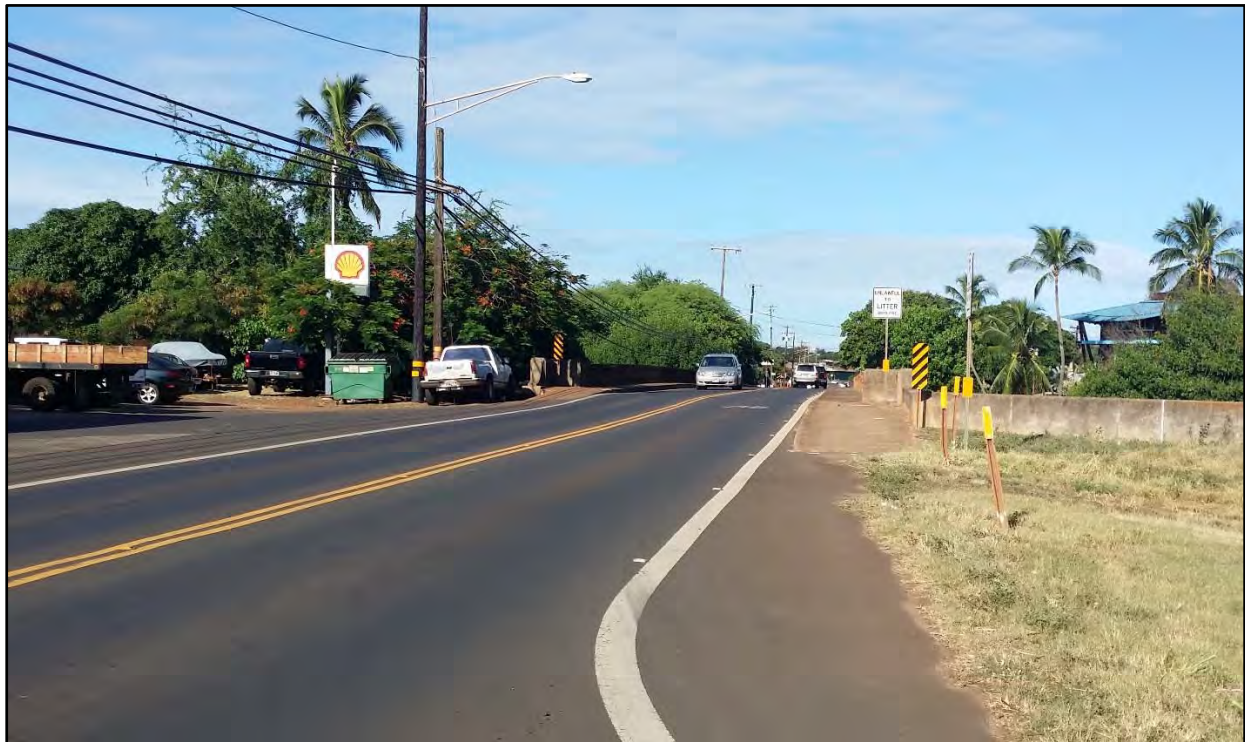
Figure 33. Kaumuali'i Highway extending over Hanapēpē River Bridge, view to west
