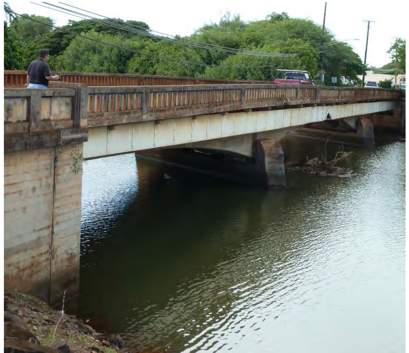
Photo 1: Mauka side of Hanapepe River Bridge, looking west
