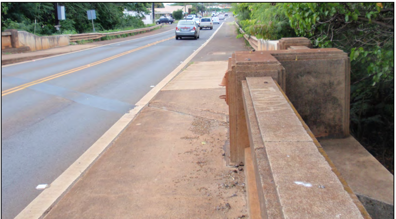
West end of Hanapepe River Bridge, looking west.
