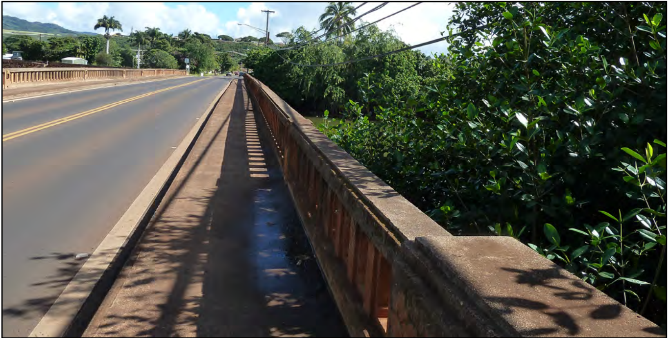
Deck of Hanapepe River Bridge, looking east.
