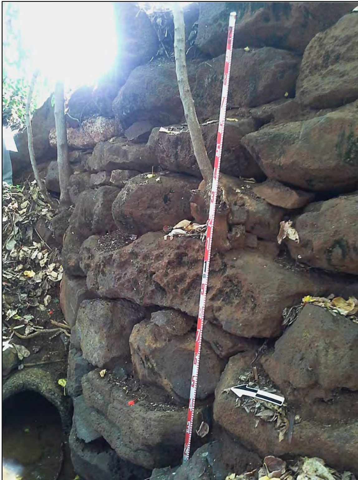
Figure 46. North end of SIHP # -2282, retaining wall, view to northeast
