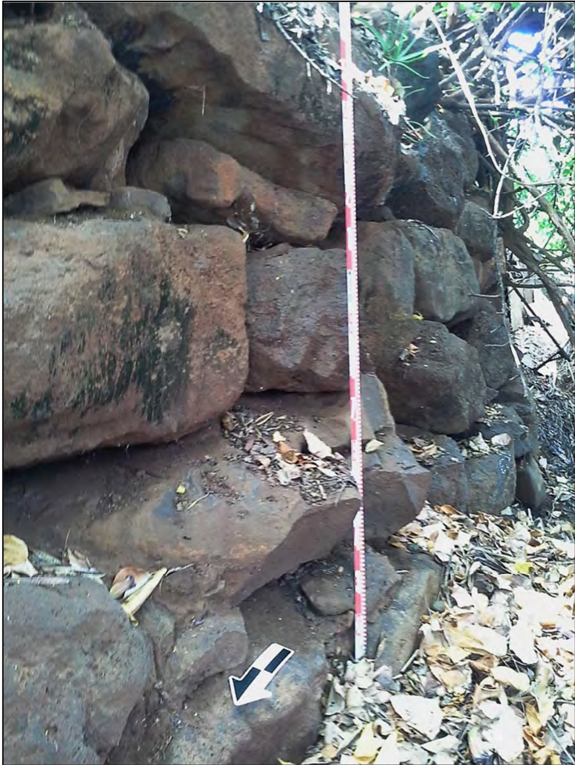
Figure 45. Central portion of SIHP # -2282, retaining wall, view to north
