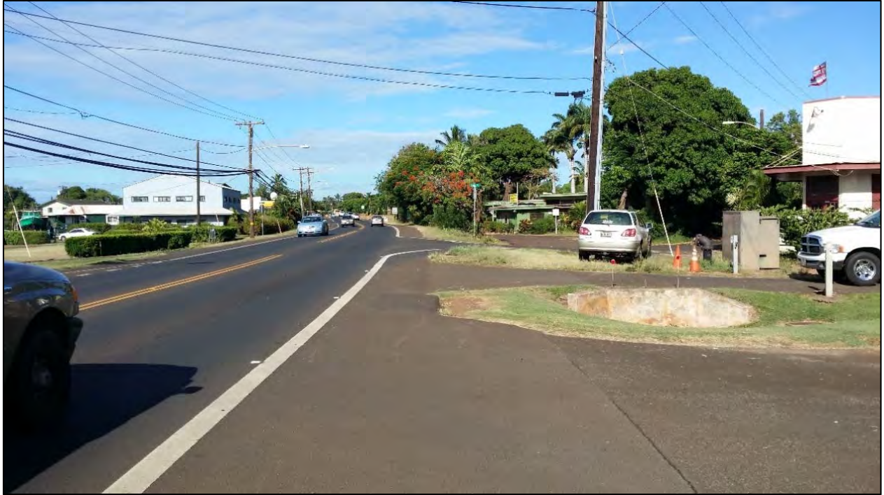
Figure 6. General view of the project area on the east side of Hanapēpē River Bridge showing Kaumuali'i Highway, view to west
