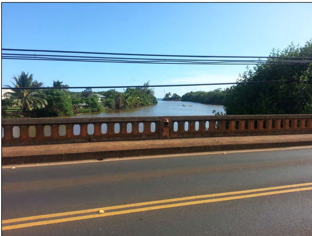
Figure 6. Hanapēpē River looking downstream of the bridge toward Hanapēpē Bay.
