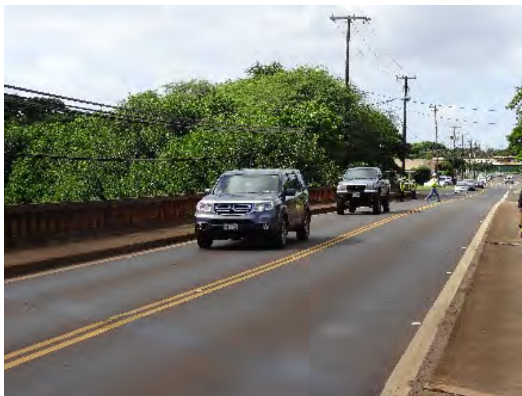
Photo 2: View of Hanapepe Bridge looking west
