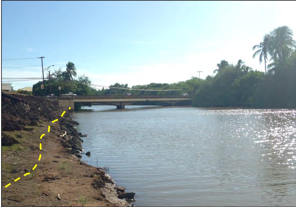
Figure 5. Hanapēpē River bridge, showing modifications on the right bank. Note: high tide line is shown by yellow lines.
