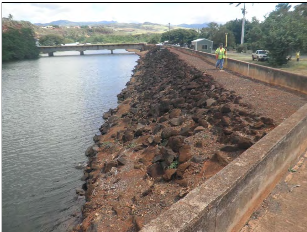
Figure 51. SIHP # -2283, floodwall, view to north
