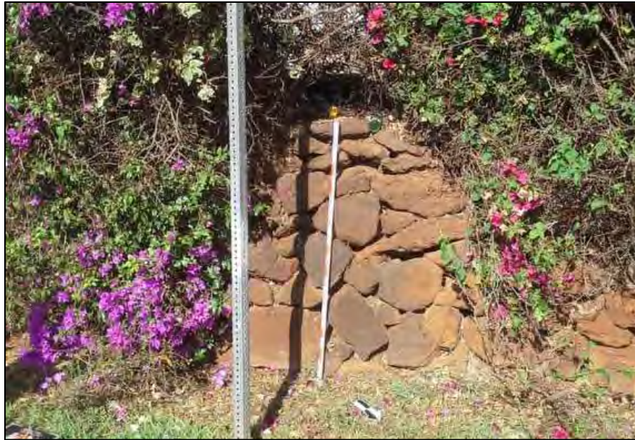
Figure 54. SIHP # -2284, retaining wall, view to southwest
