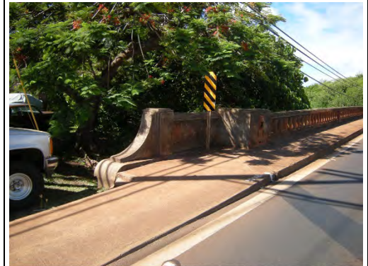
Hanapepe River Bridge, view facing west
