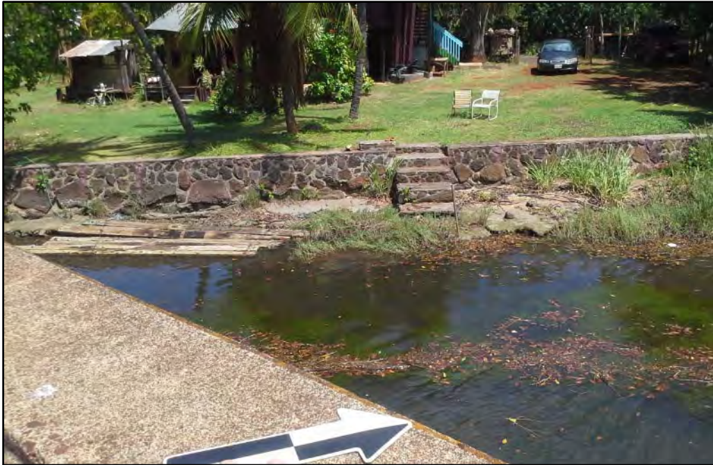
Figure 34. SIHP # -2281, retaining wall lining Hanapēpē River, view to northwest
