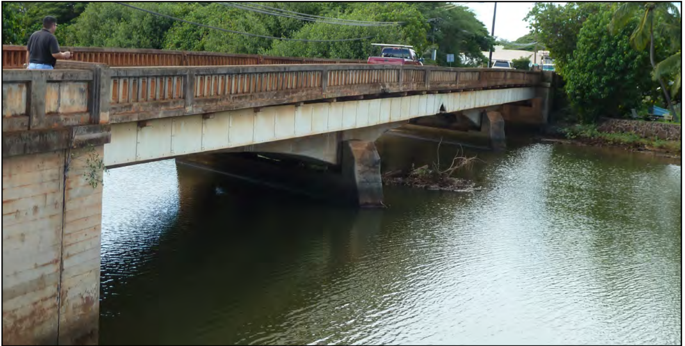
Upstream side of Hanapepe River Bridge, looking west.
