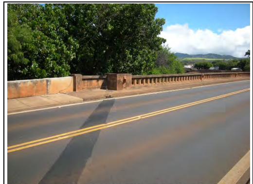
Hanapepe River Bridge, view facing northeast
