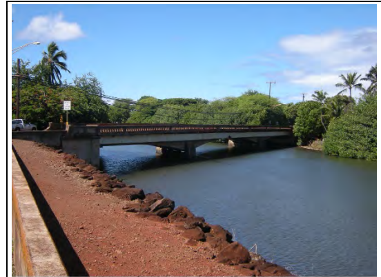
Hanapepe River Bridge, view facing south
