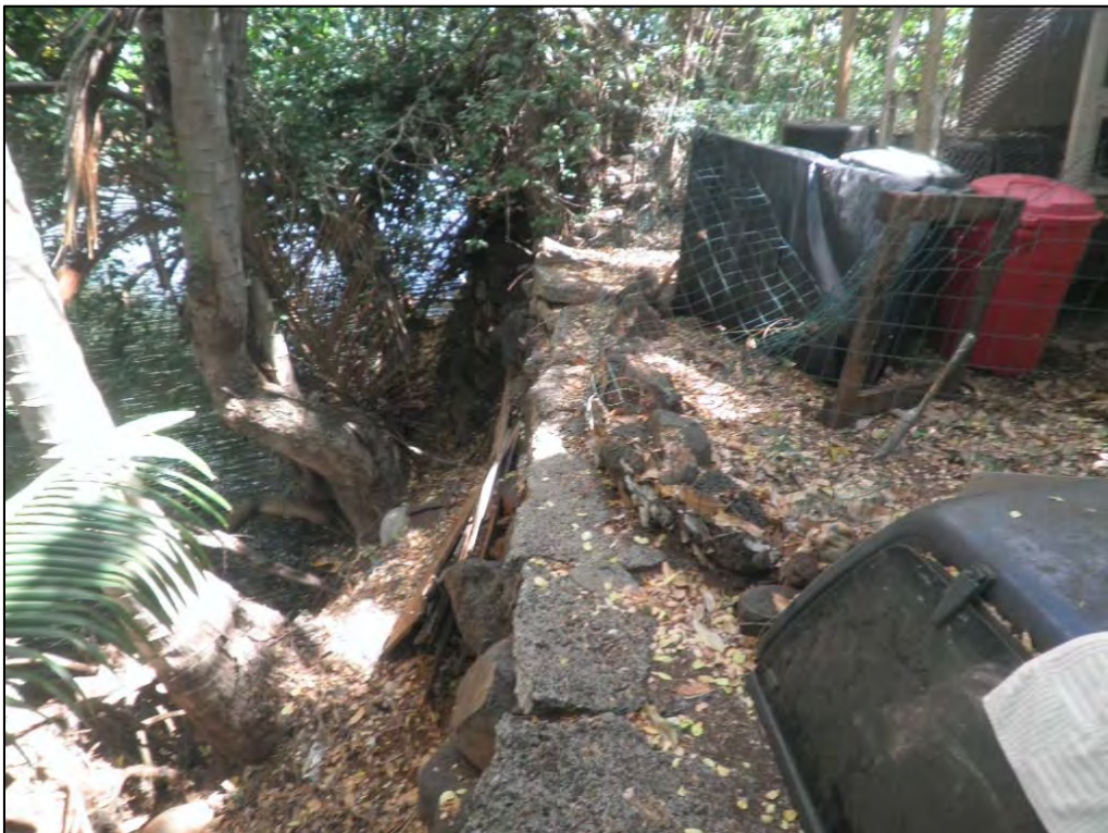
Figure 42. SIHP # -2282, retaining wall, view to north
