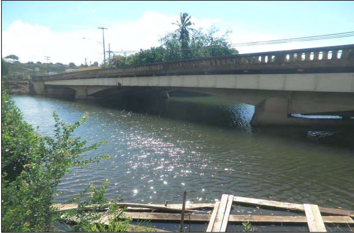
Figure 32. SIHP # -2280, Hanapēpē River Bridge, view to southeast
