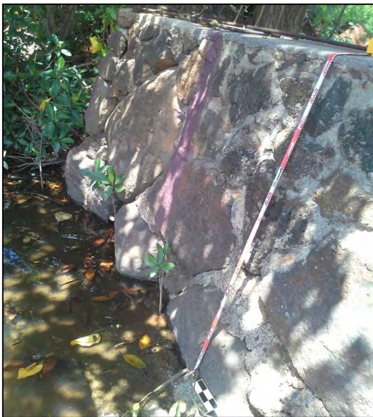
Figure 35. South end of SIHP # -2281, retaining wall, view to west
