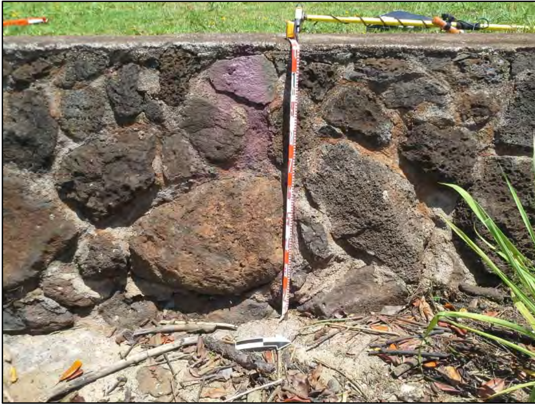
Figure 36. SIHP # -2281, retaining wall, view to north
