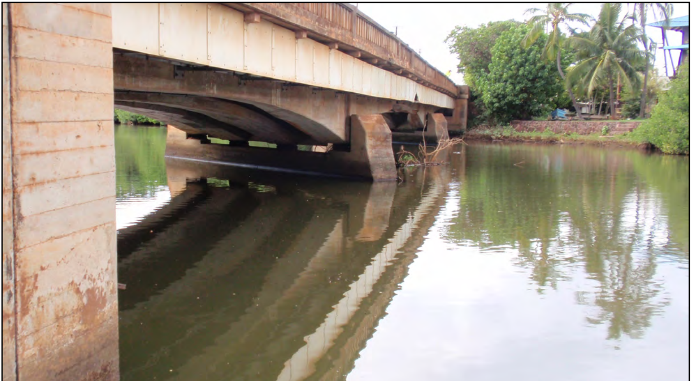
Substructure of Hanapepe River Bridge, view from east bank.
