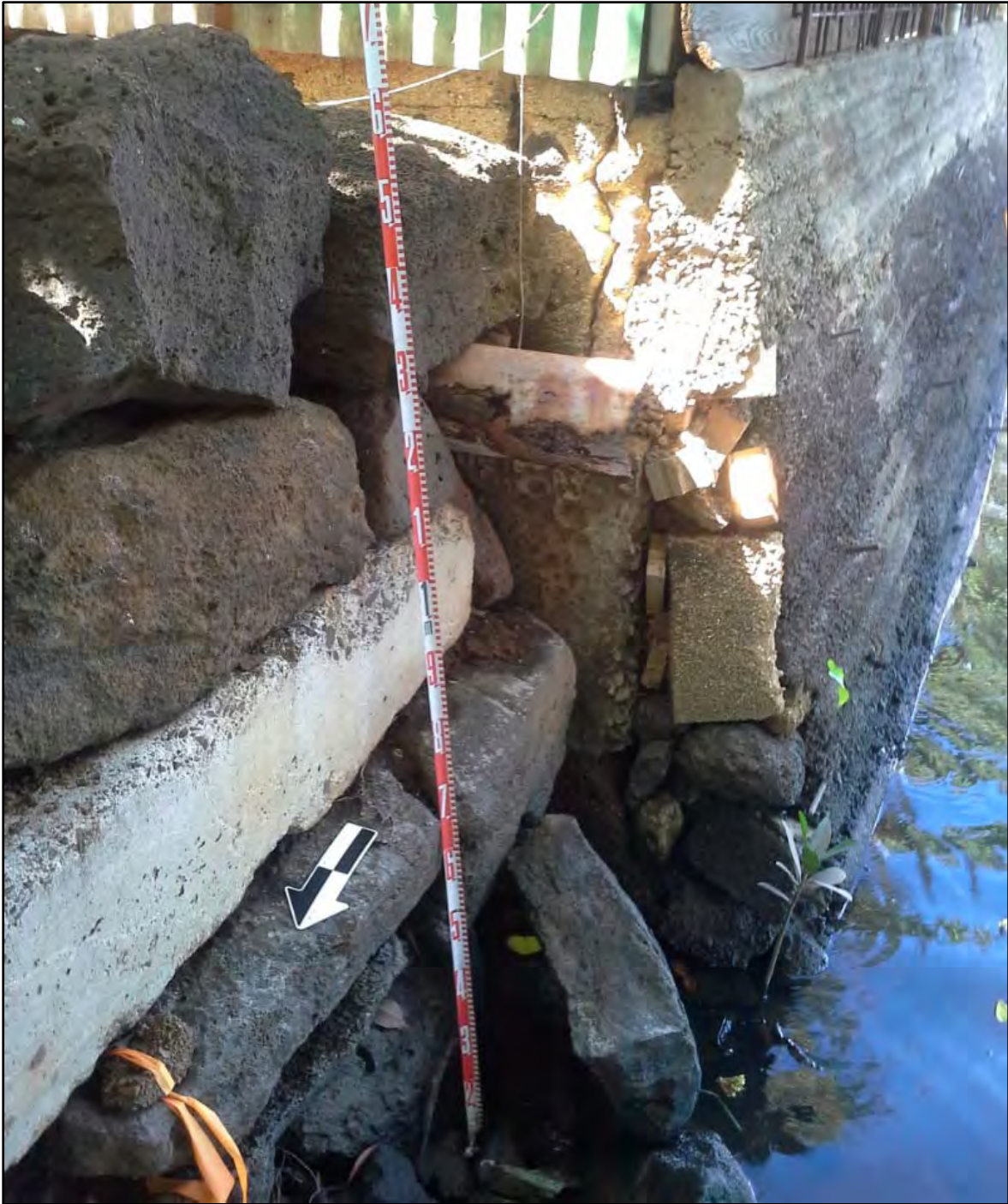
Figure 44. South end of SIHP # -2282, retaining wall, view to south
