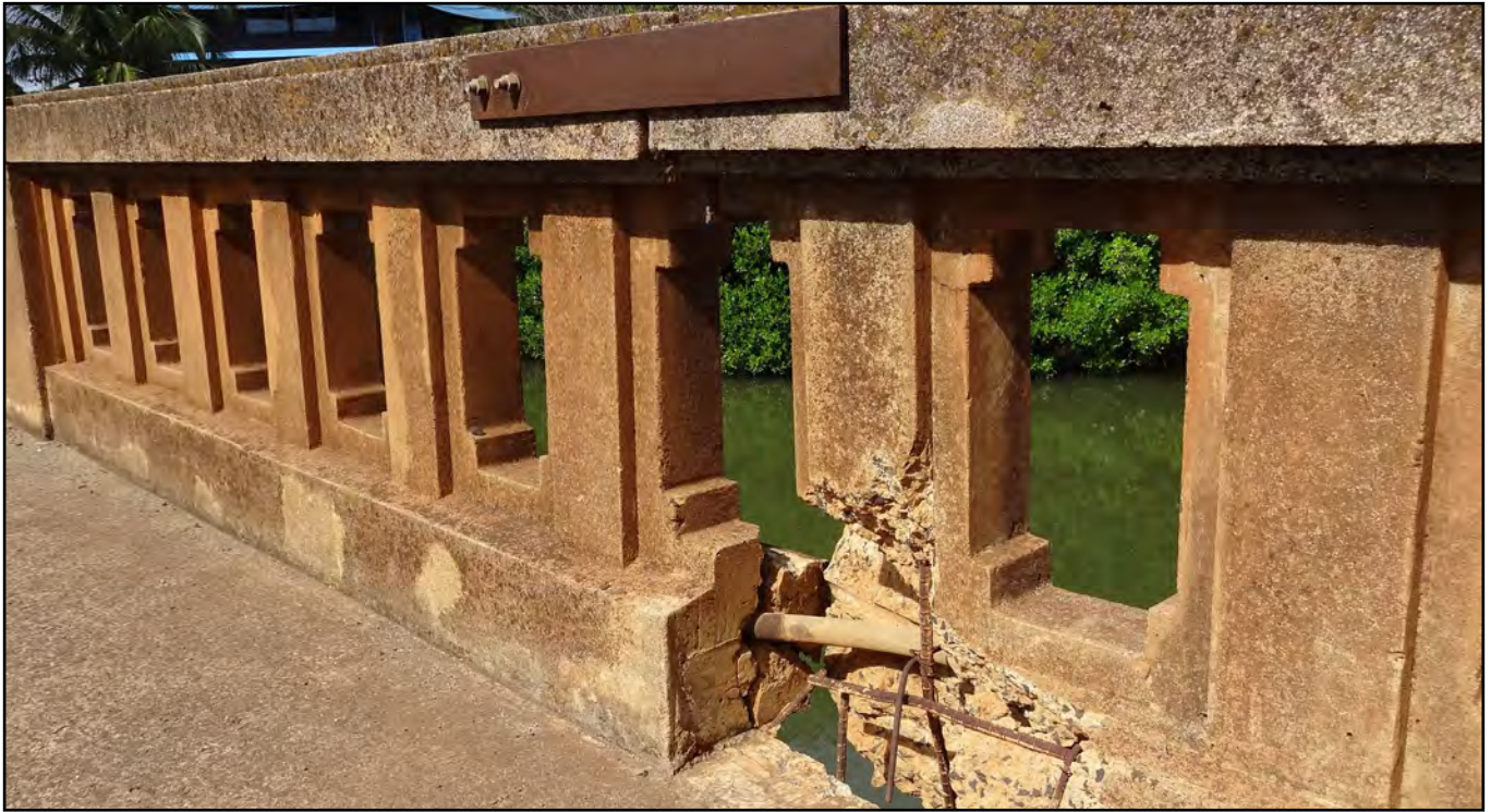
Bridge railing close up.
