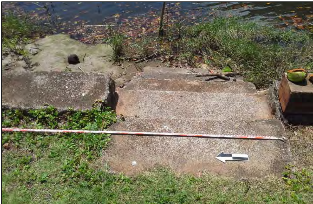
Figure 39. SIHP # -2281, stairs leading from the residential property into Hanapēpē River, view to east
